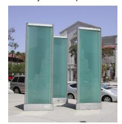
long time. The restoration will involve a thorough inspection and, as necessary; repair of all components (including the electric gear motors); replacement of the existing metal halide lights with longer-lasting and more energy efficient LED bulbs; and a thorough cleaning and resealing of the glass on each of the three pillars. Restoration will take approximately one month to complete, with the majority of the work taking place off-site.
