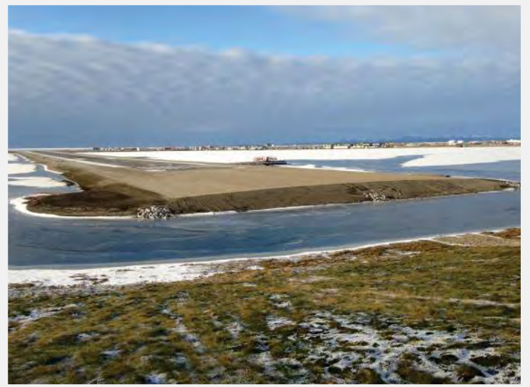
Kotzebue Airport - view of new runway safety area constructed on runway east end.
