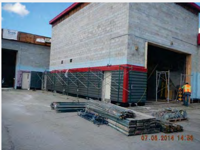
ARFF building at FAI was rehabilitated in 2014
