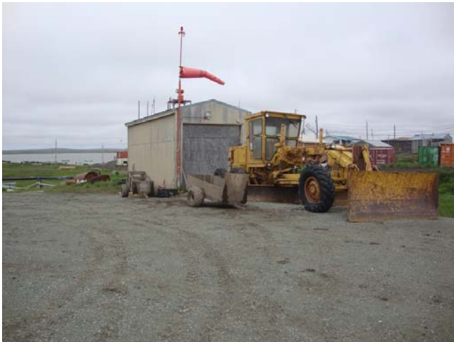
Kipnuk's snow removal equipment building and grader.
