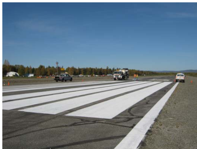
Runway maintenance at the airport includes crack sealing, paving, painting and lighting repair.
